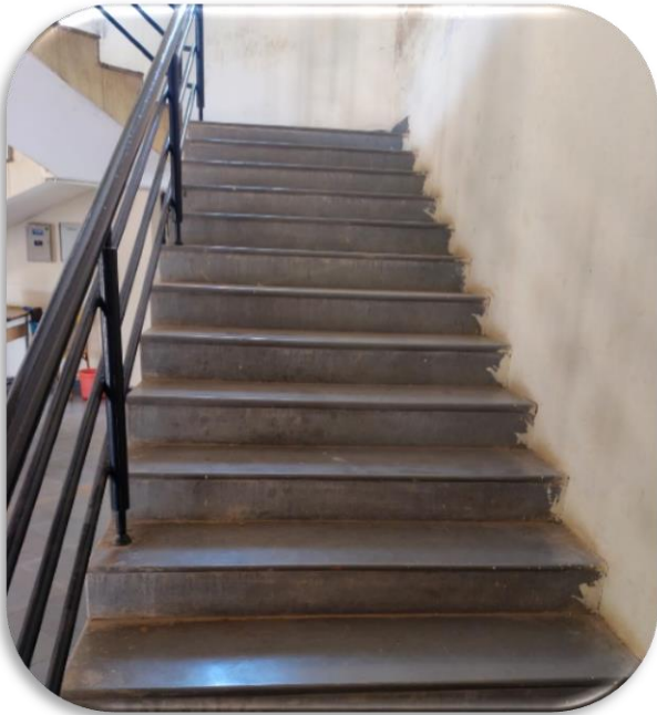
Wide-well ventilated staircase
