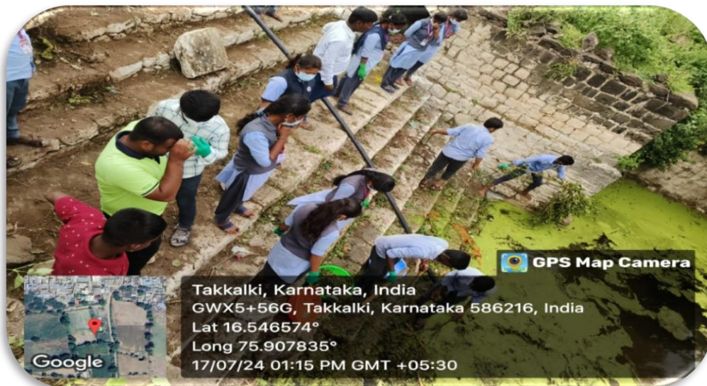
Cleaning of open well
